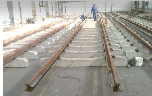
Grooved profile Spurrillenschiene 49E1 pre- assembled in Pražská strojírna a.s. on concrete sleepers and installed in Prague
