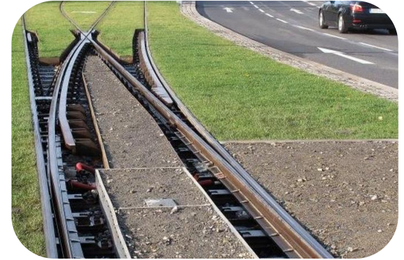
Flat bottom LRT turnouts - T rail
