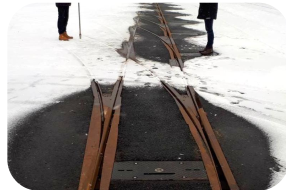
heating the switches
