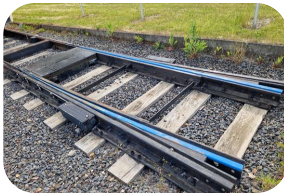
switch with flexible blades
