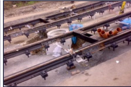
Installation of drainage boxes into gauge
