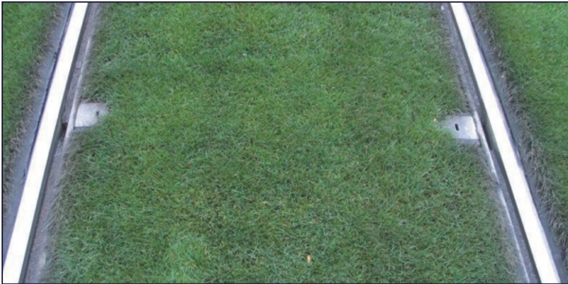
Solution for tracks where drainage is embedded into a grass layer
