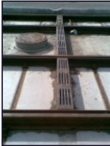
Drainage of tram track before application of tarmac cover
