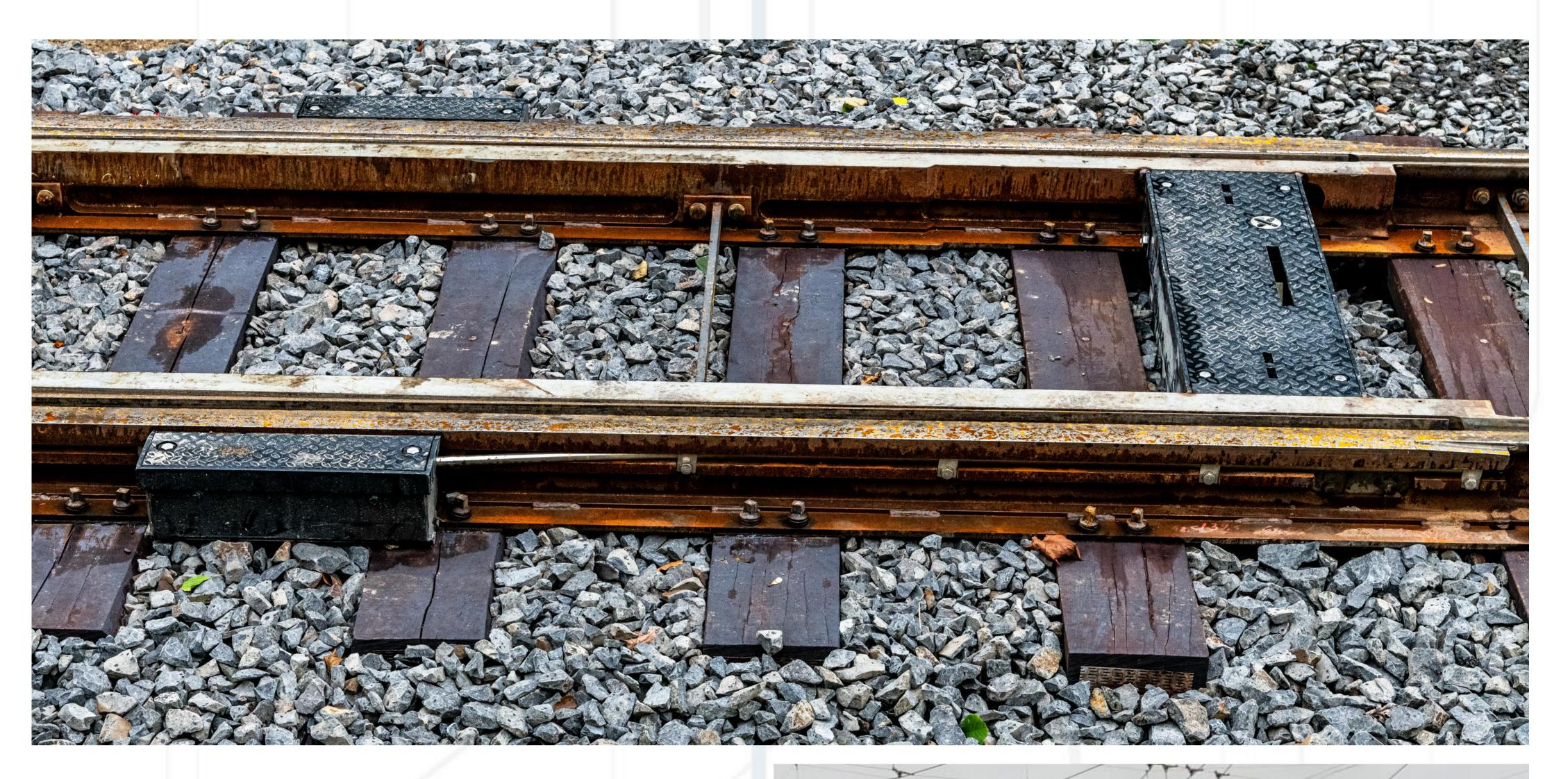
The device is used to heat switches with flexible or pivot tongues to ensure their proper functioning at air temperatures below freezing and in adverse weather conditions (icing, snowfall). The heating can be operated either as unregulated (direct switching on and off of the heating) or as regulated depending on the outdoor temperature. The direct or regulated heating function can be selected by setting the heating mode in the switch control system.
